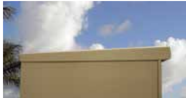
Sloped top for moisture runoff
